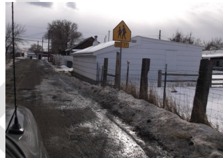
Figure 6: Building restricting the availability of sidewalk placement on the west side of Piccolo Lane
